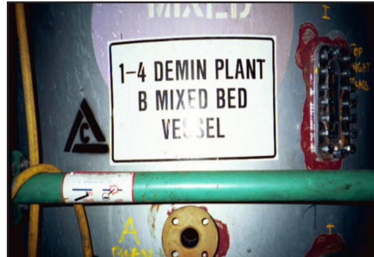
External view of the tank
