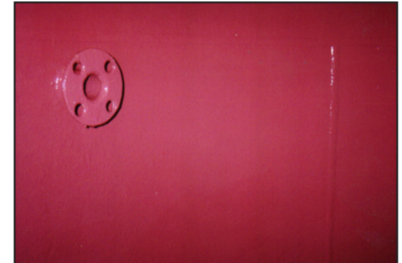
After proper surface preparation, ARC S4+ was applied in a two-coat system
